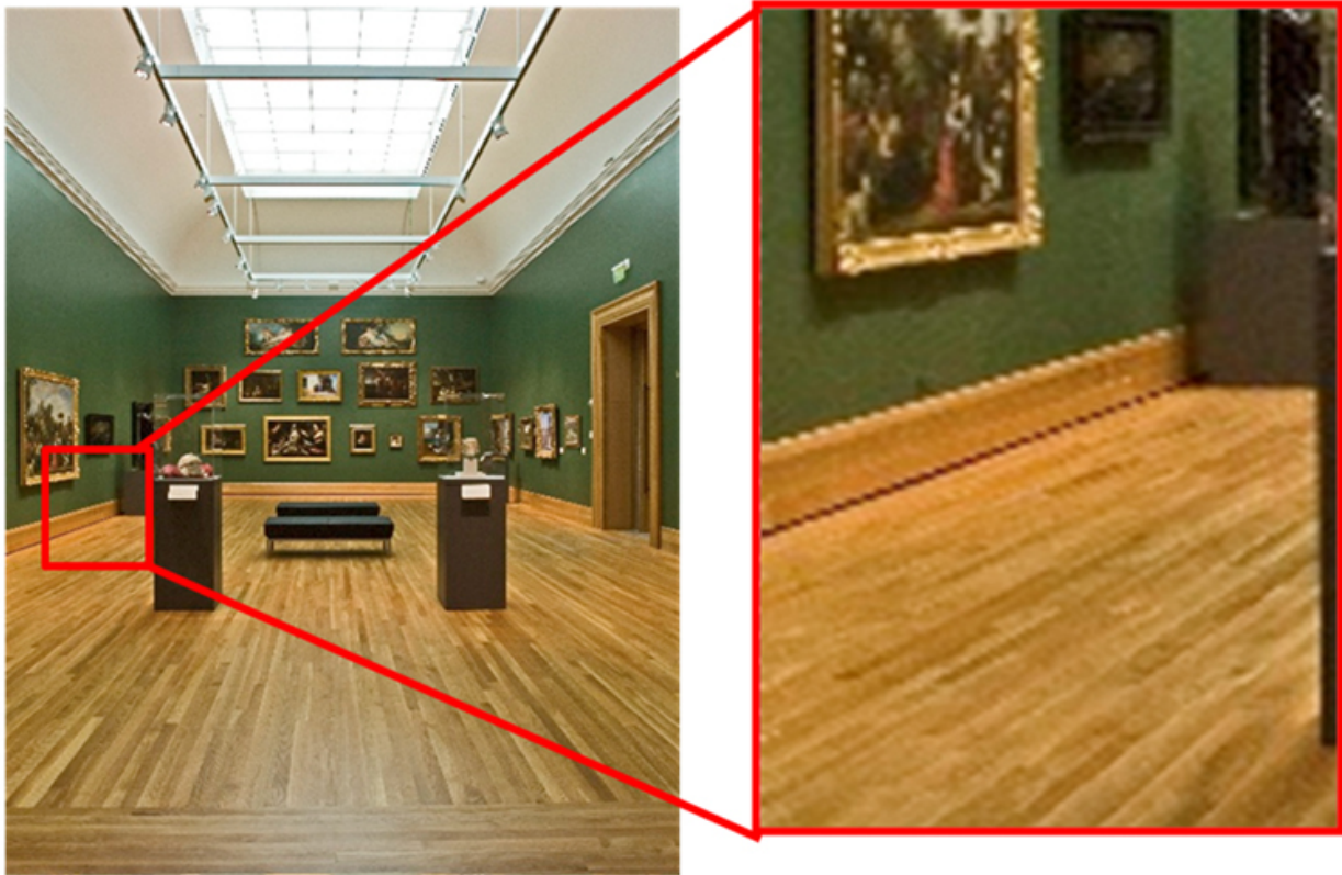
Photo 7 – Vented wall system installed in finished gallery space.
