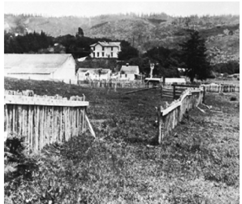
This picture, taken in Marin County, CA (1906) shows a fence that was offset about 8.5 feet along the trace of the fault
