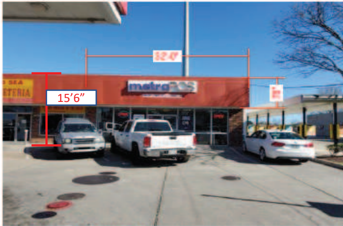
PHOTO SURVEY OF EXISTING
