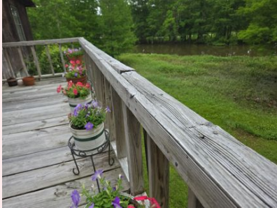
Weather worn and warped materials which are starting to pull the nails loose and extending The cracking around the nails making them less effective
