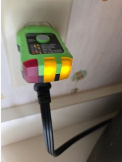
Kitchen electrical at time of inspection.
