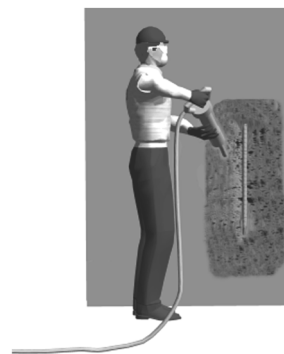
Unsound concrete removed with 15-lb chipping hammer. Hammers larger than 15-lb class may cause damage to substrate and reinforcement.
