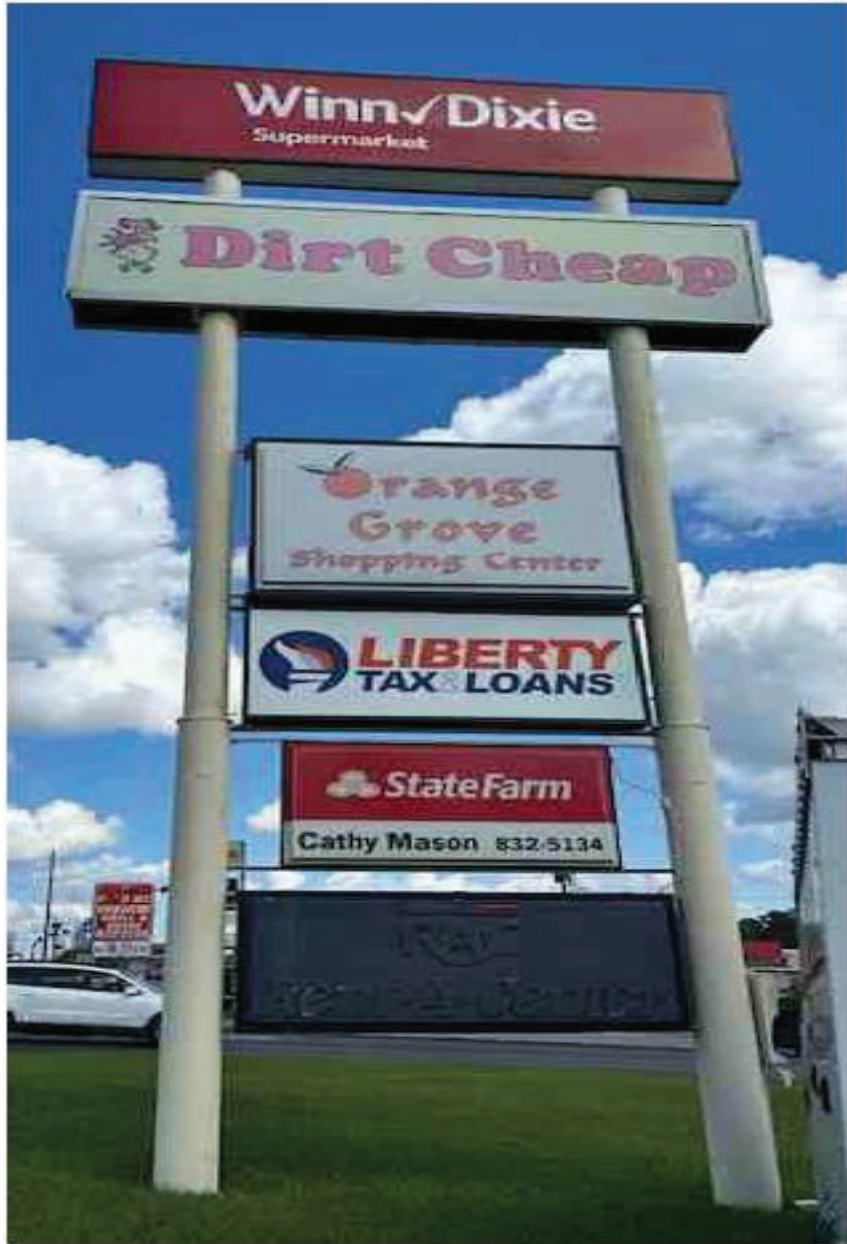
EXISTING 5'-1" X 10'-0 1/2" PYLON 2" RETAINER
