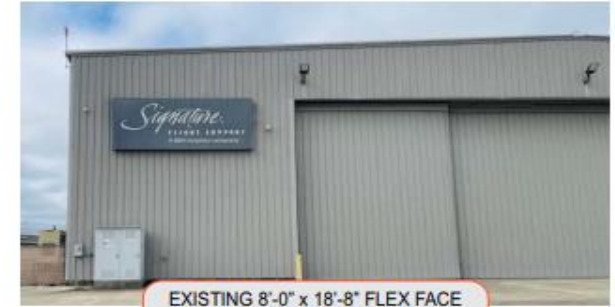
EXISTING 8'-0" x 18'-8" FLEX FACE TO BE REMOVED & REPLACED
