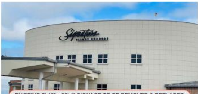
EXISTING 5'-10" x 20'-1" SIGNAGE TO BE REMOVED & REPLACED WALL TO BE REPAIRED AS REQUIRED
