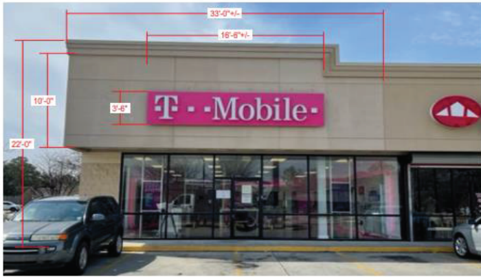
PHOTO SURVEY OF EXISTING
