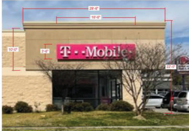
PHOTO SURVEY OF EXISTING
