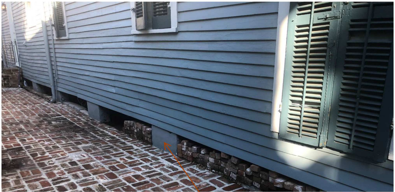
Piers Supporting Residence
