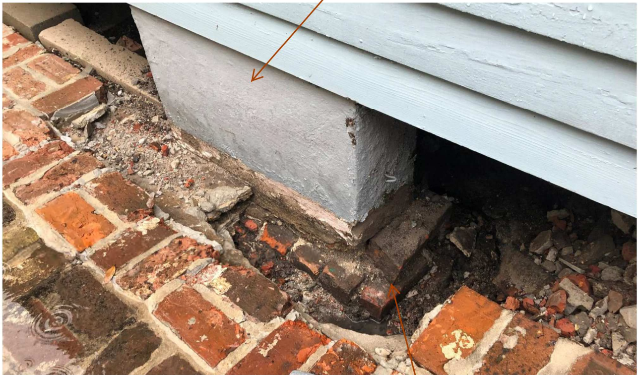
Foundation Supporting Piers
