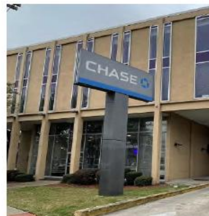
EXISTING CONDITION - NOT TO SCALE - REMOVE AND REPLACE W/ NEW M-12-RE
