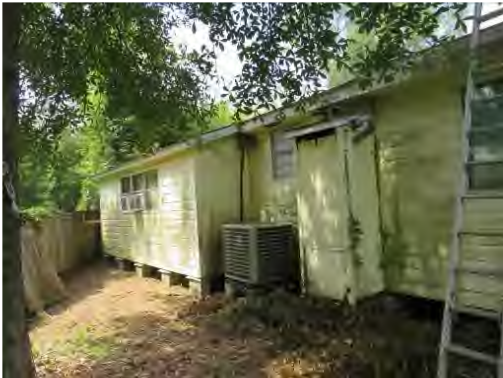
Photo No. 4: East (right) elevation of residence.
