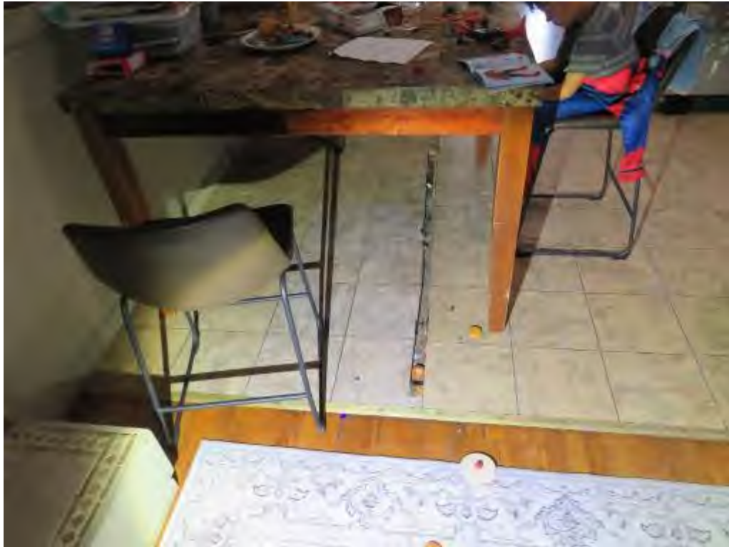
Photo No. 29: The wood planks extended under the kitchen's floor tiles.
