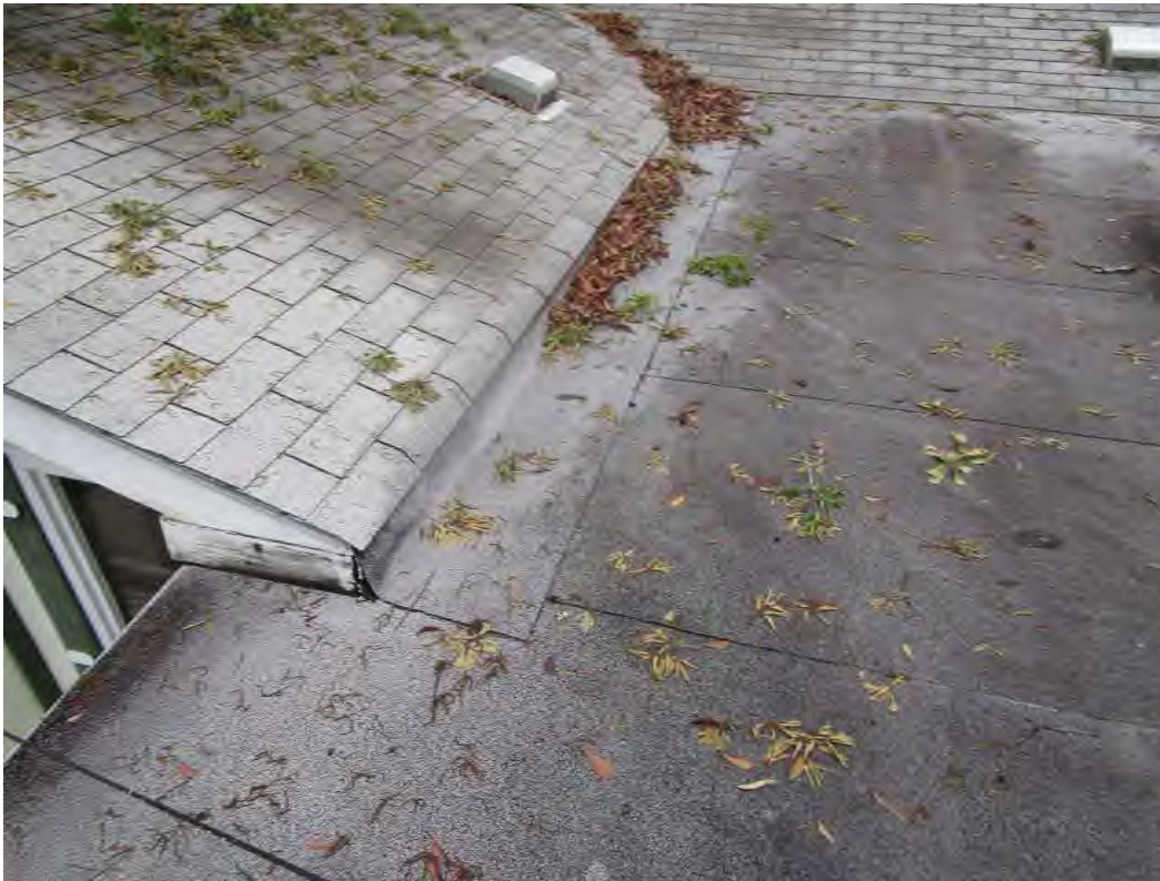
Dwelling/Front Flat Roof - 21-
