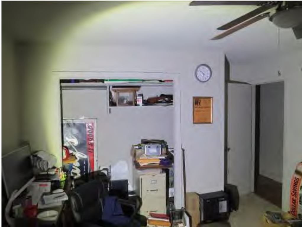
Photo No. 31: No stains were noted on the bedroom's ceiling or walls.
