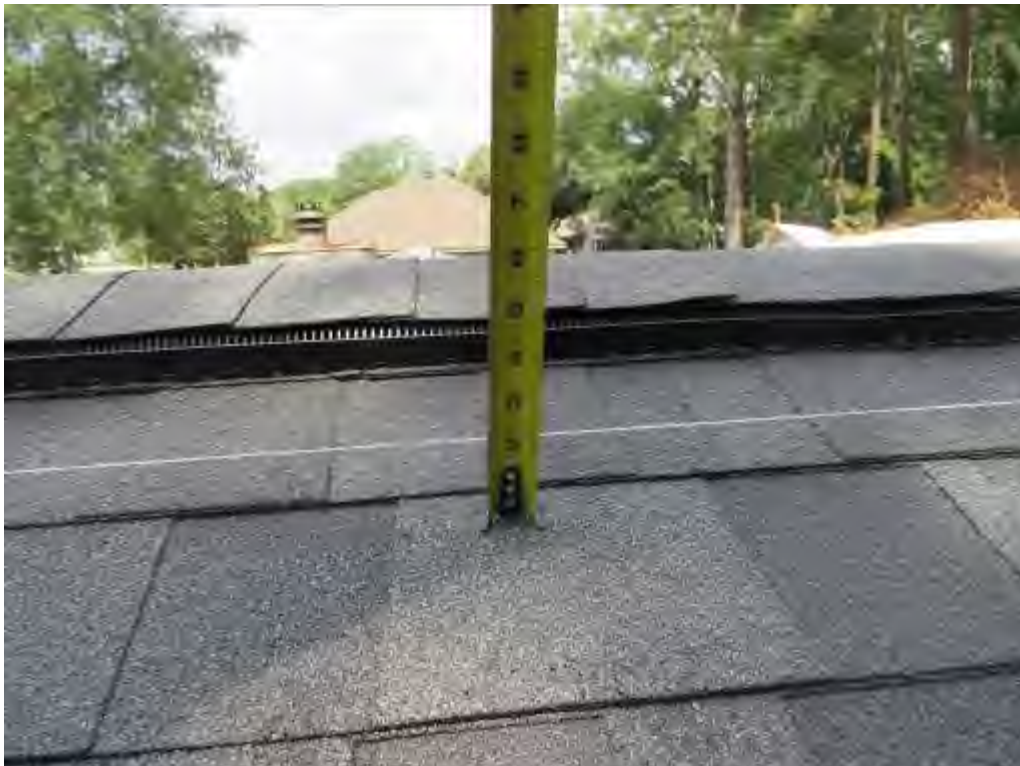
Photo No. 14: Low-point at north-side ridgeline.
