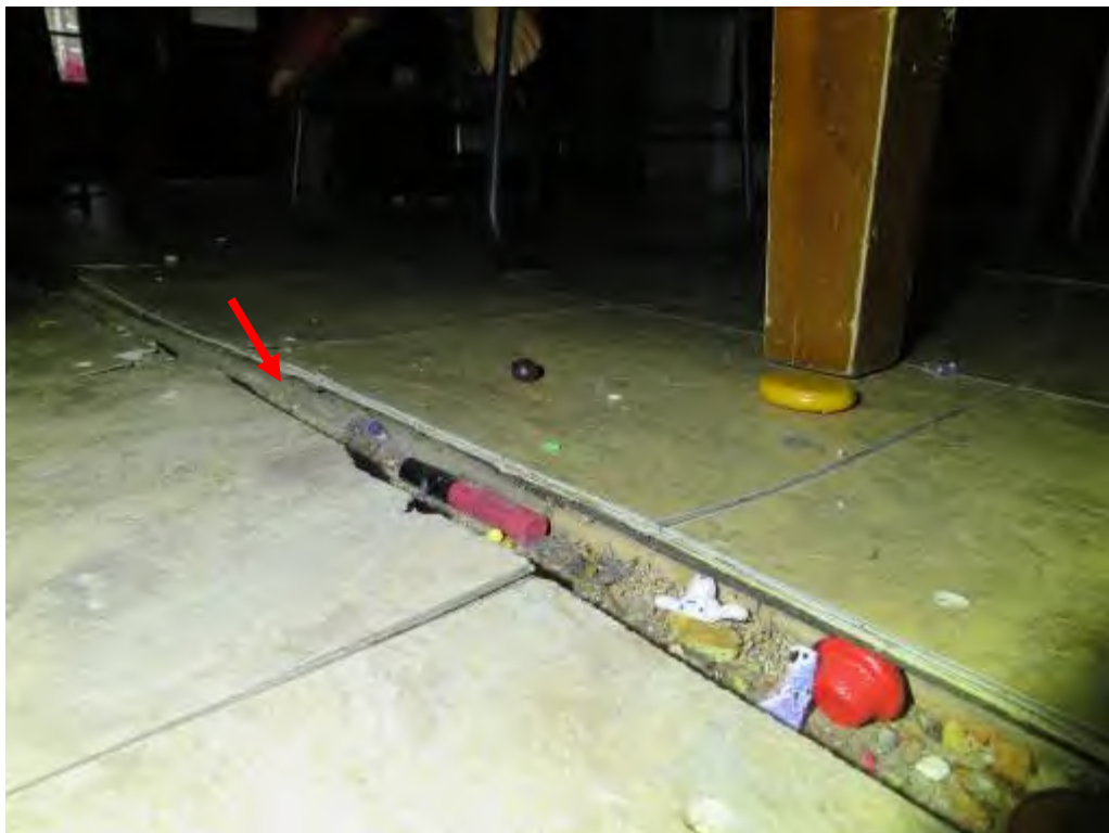
Photo No. 24: The hardwood flooring was dark in color.
