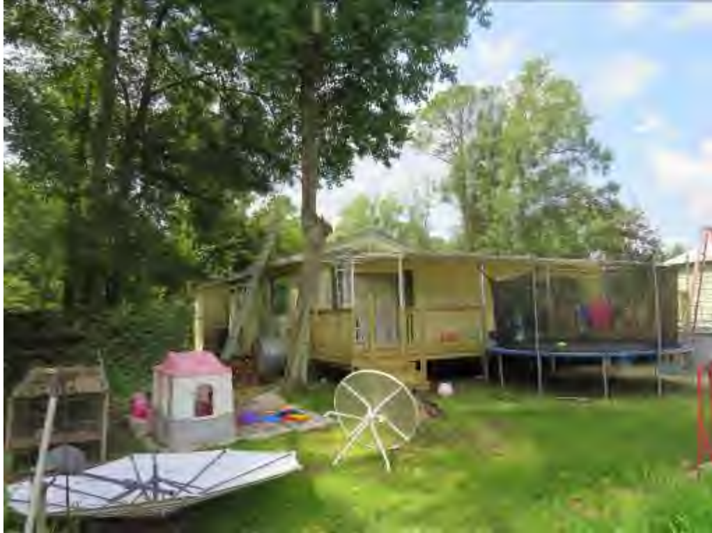
Photo No. 5: North (rear) elevation of residence.
