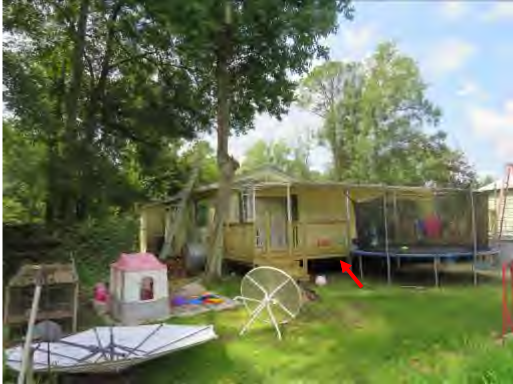
Photo No. 9: The rear porch appeared recently constructed.
