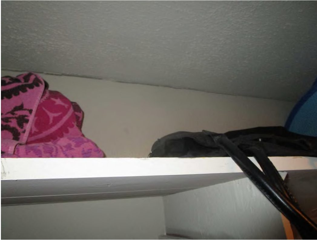
Interior/Rear Bedroom Closet - 61-
