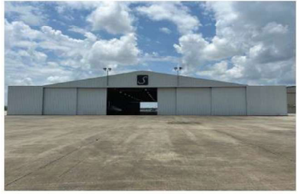
EXISTING FACE TO BE REMOVED & REPLACED
