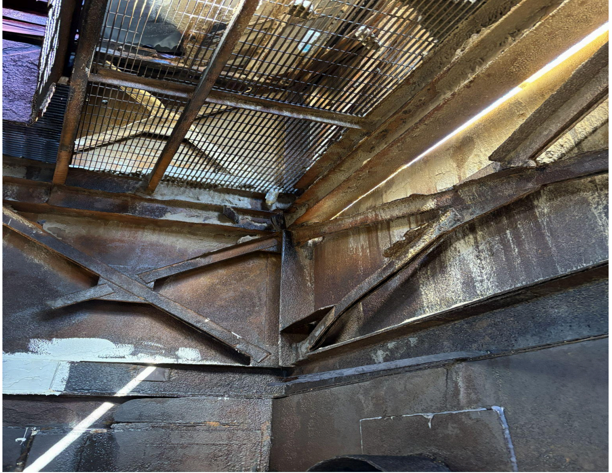
(Photo C) interior view level two looking northwest
