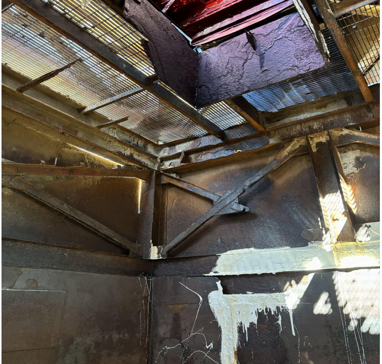
(Photo D) Interior view level 2 looking southwest
