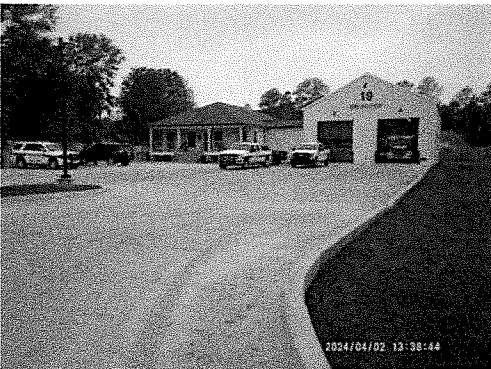
St. Tammany Fire Protection District #1 New Apparatus bay & Living Quarters 2023
