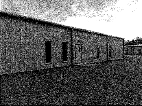
St. Tammany Fire Protection District #1 New Training Facility 2024
