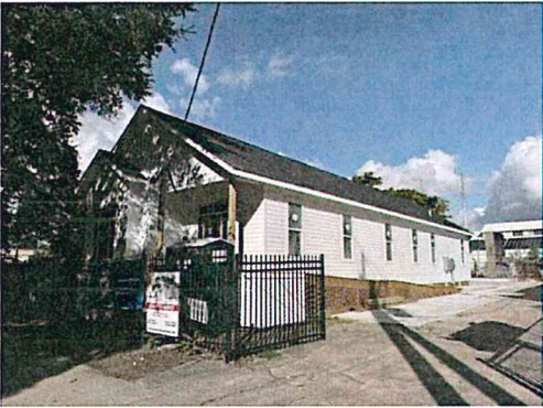
New Dental Office NOLA Under Construction 2024
