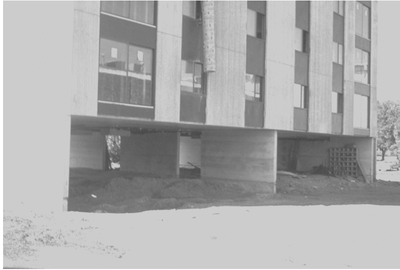
Figure 5-9: Building elevated on parallel stem walls.
