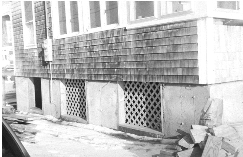
Figure 5-10: Building elevated on crawlspace with openings.
