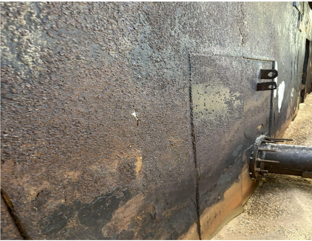
(Photo A) Exterior view level one looking northeast
