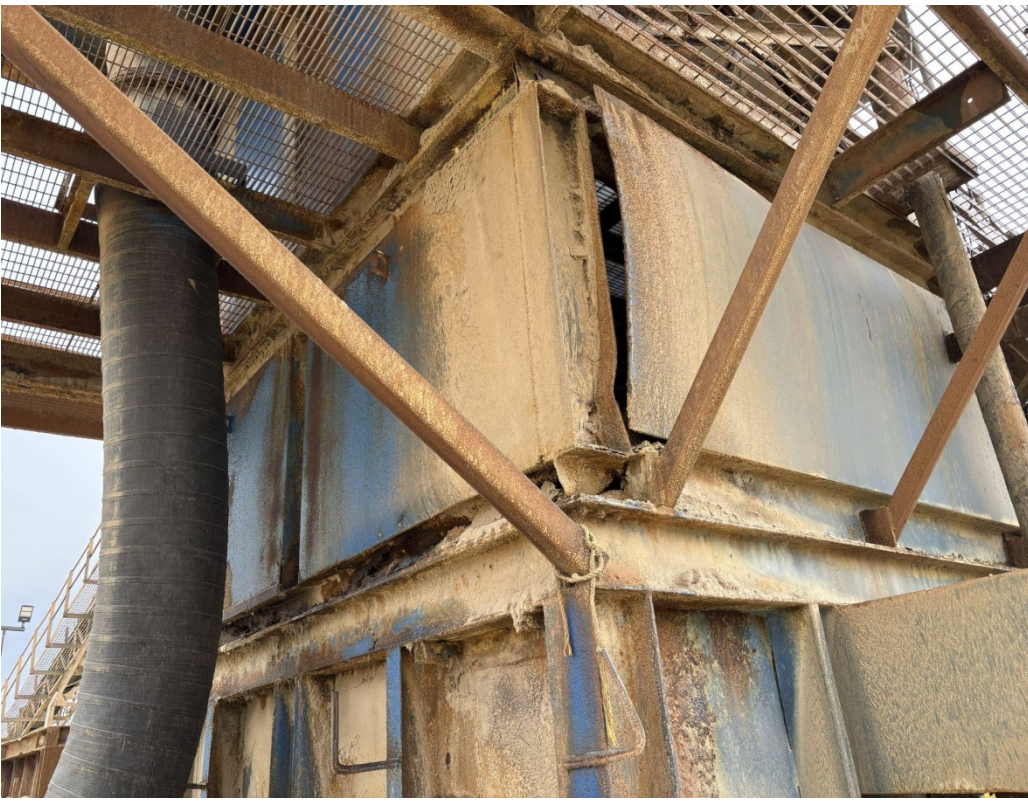
(Photo E) exterior view level 2 looking north east
