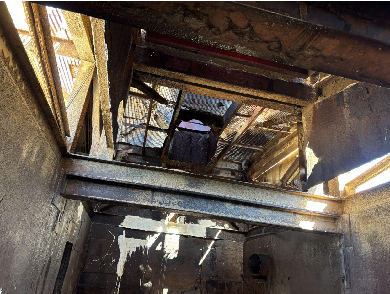
(photo B) Interior view level 1 under vibrator screen looking west
