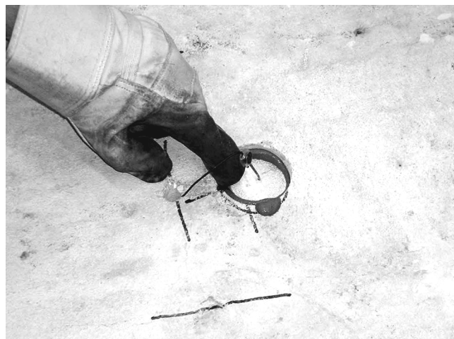
Fig. 13—Anode placed in hole with patching material.
