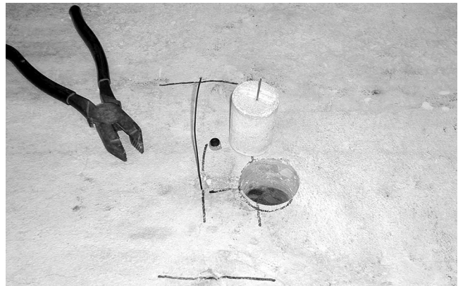
Fig. 11—Secondary hole with reinforcing steel connection.
