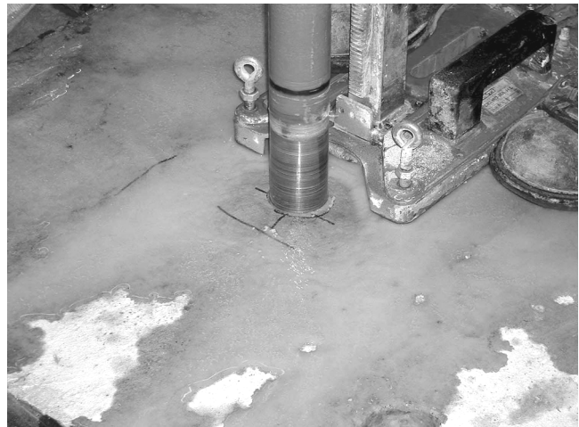
Fig. 10—Coring hole for anode.
