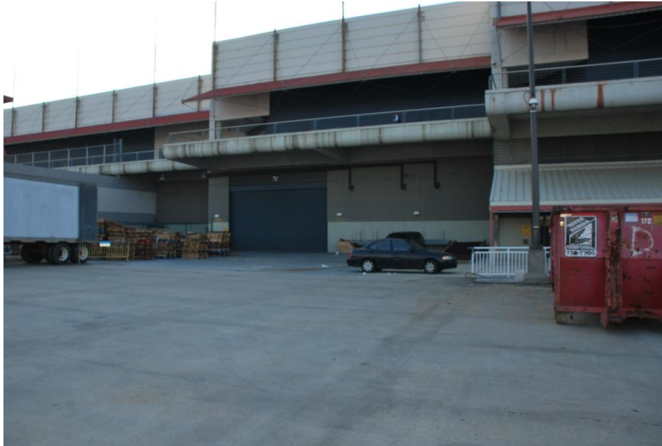
Exterior of the riverside of existing Julia Street Cruise Terminal with cruise ship service trucks.
