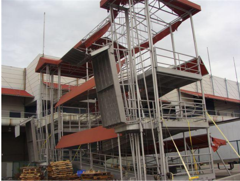
Existing inferior switchback gangway at the Julia Street Terminal.
