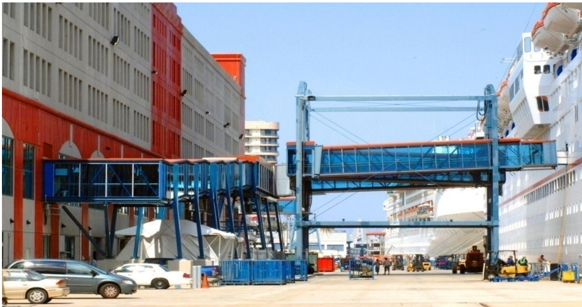
Elevated, enclosed, climate-controlled articulated passenger gangway at the Erato Street Cruise Terminal, adjacent to the Julia Street Cruise Terminal.
