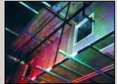
Grease Duct drywall enclosure
