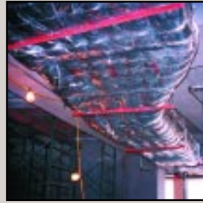
Zero Clearance to Combustibles Protection
